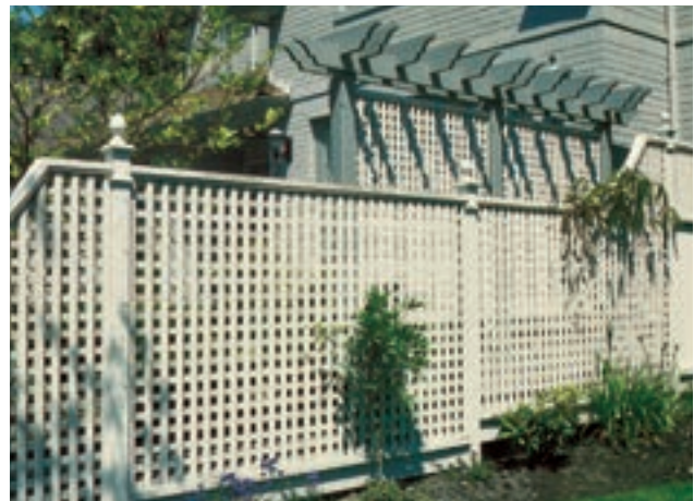
A simple post and rail lattice fence. Finials on posts add a distinctive touch.
